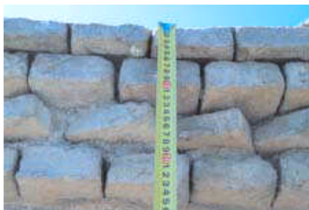
14. Fethiye mosque of Nafpaktos, a detail of the walls' stone cornice
