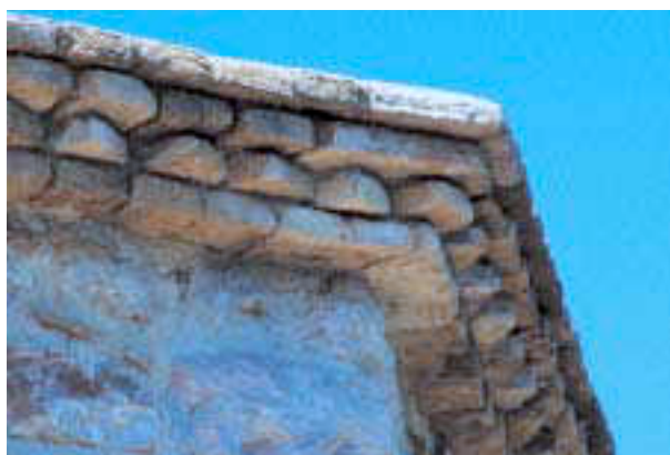
13. Fethiye mosque of Nafpaktos, a detail of the walls' stone cornice
