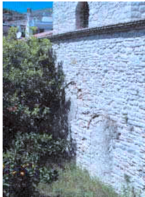
17. Fethiye mosque of Nafpaktos, a detail of the SW façade, shows the walls' construction and the walled up windows
