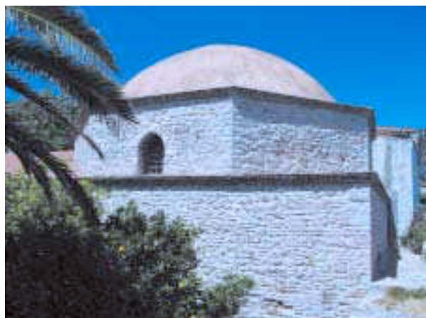
9. Fethiye mosque of Nafpaktos, the exterior gradual form; square, octagon and dome
