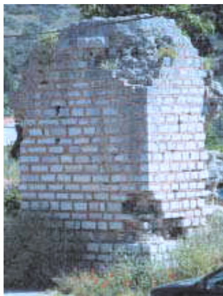
37. Vizir mosque of Nafpaktos, minaret's base, cloisonné masonry
