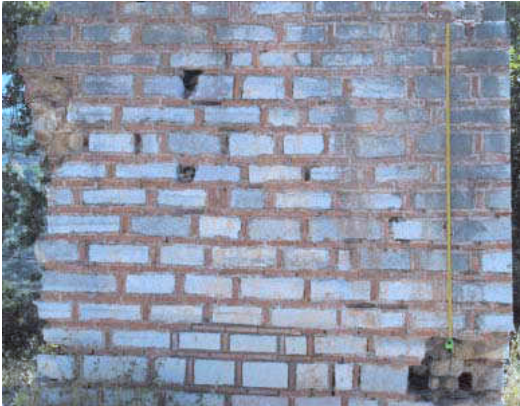
39. Vizir mosque of Nafpaktos, minaret's base, the western side; a detail that shows its cloisonné masonry according to the Byzantine Helladic School
