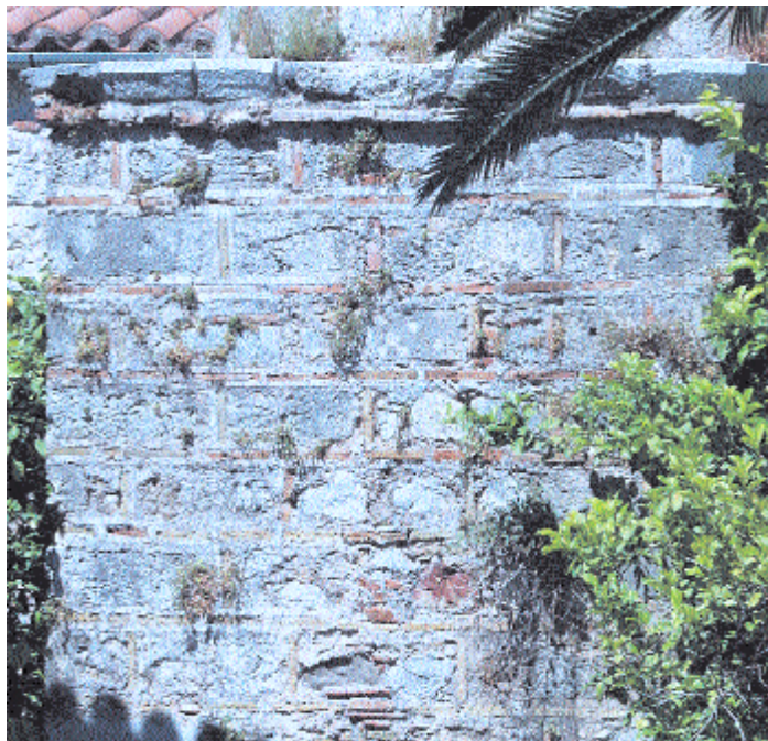
16. Fethiye mosque of Nafpaktos, a detail of the minaret's building technique "cloisonné"
