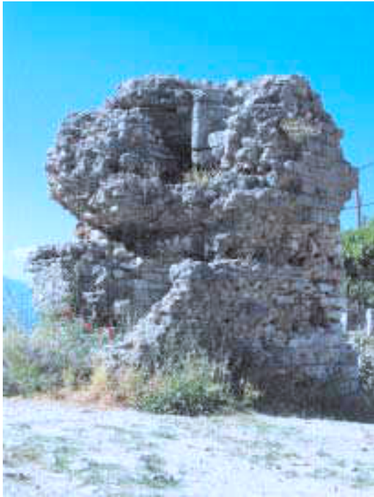
27. Vizir mosque of Nafpaktos, minaret's base, its door, a ruined spiral staircase
