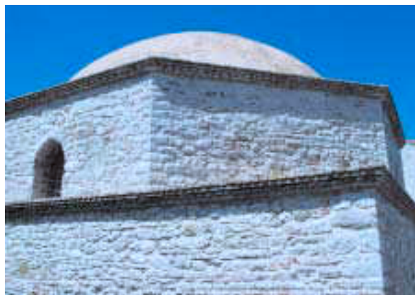
12. Fethiye mosque of Nafpaktos, a detail of the walls' construction with their cornices and the windowed drum
