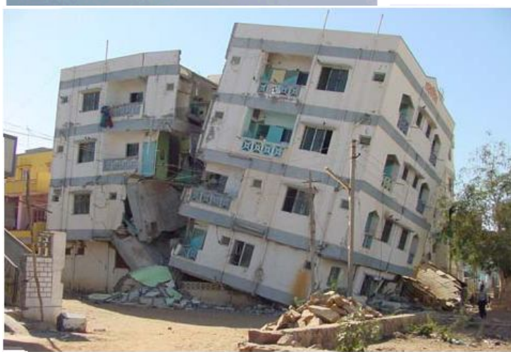
Collapse of reinforced concrete columns (and building) during 2001 Bhuj (India) earthquake
