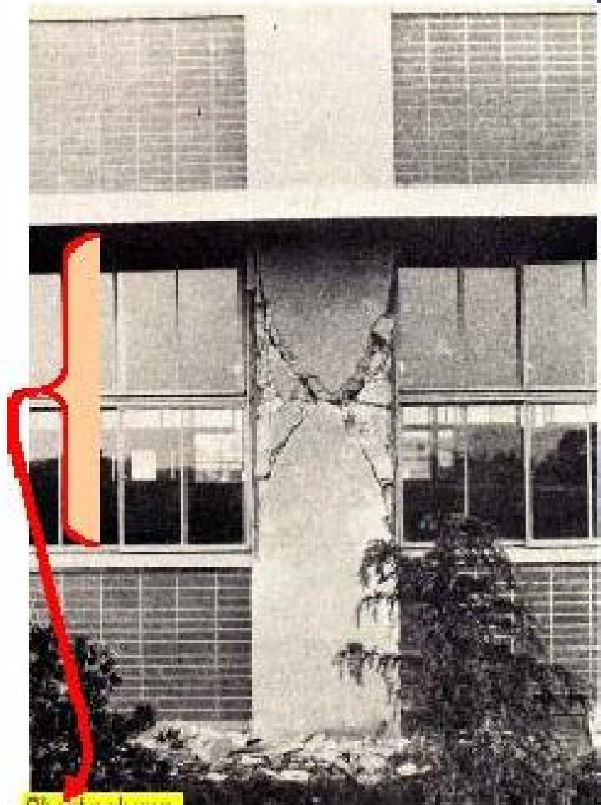
Short column between lintel and sill of window
