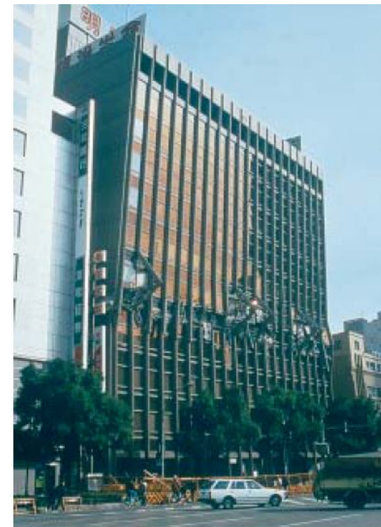
5/2 In this office building also, an upper storey failed. The top of the building has collapsed onto the floor below, the whole building rotated and leaned forwards.
