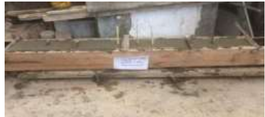
Fig. 3. Casting of Beams
